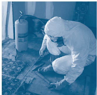
Wet the Floor Before, During, and After Removal
