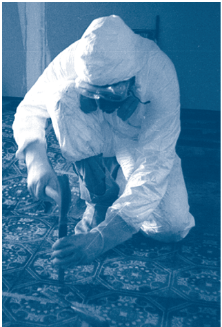
Cutting the Floor
