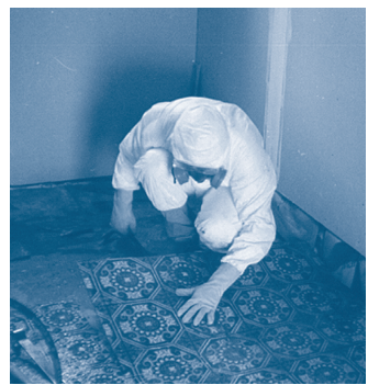
Lift and Peel up Flooring
